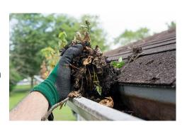
An accumulation of debris that is not taken care of can cause your gutters to crack, sag, and detach from the home. Standing water in your gutters increases the chances of rust and corrosion. If you neglect your gutters gravity will make sure that the built up water and debris will reach the ground. Unfortunately it might be a costly mistake to your wallet.
